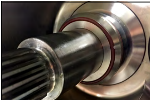
Figure 104 - Seal cap installed on shaft
